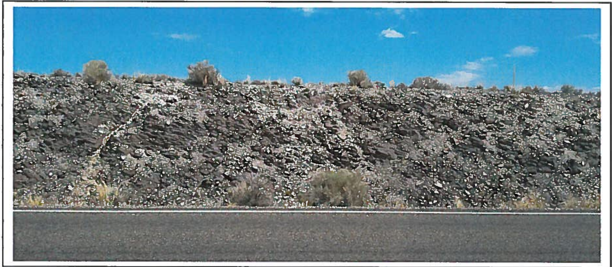
FIGURE 2 ROCK WITHIN CUTSLOPE NEAR STATION 765+00
