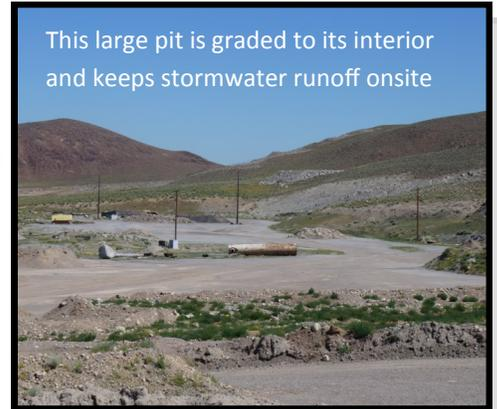
This large pit is graded to its interior and keeps stormwater runoff onsite
