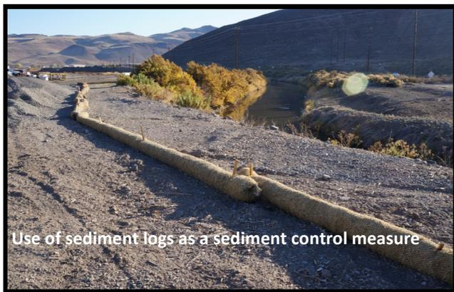
Use of sediment logs as a sediment control measure
