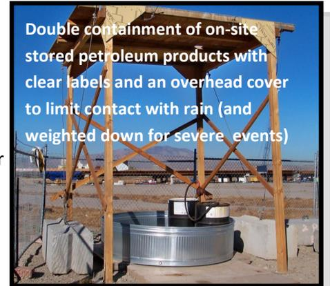
Double containment of on-site stored petroleum products with clear labels and an overhead cover to limit contact with rain (and weighted down for severe events)
