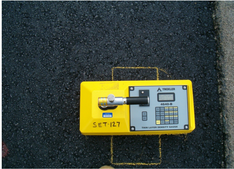
Thin layer density gauge positioning for one density test location.
