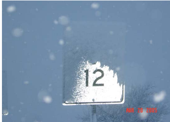
Figure 3-6. In Some Storms Even the Message of 12° Tilted Sign Cannot Be Intirely Read (Storm date 3-20-2005)
