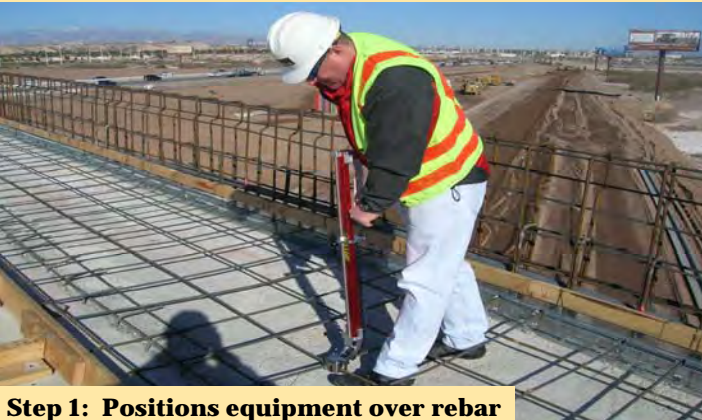
Step 1: Positions equipment over rebar
