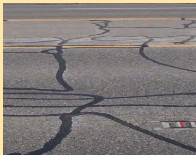
Crack Sealing
