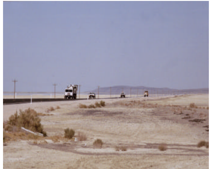
Photo 2. NDOT Ely's Striping Crew Places Waterborne Pavement Markings on US 50.
