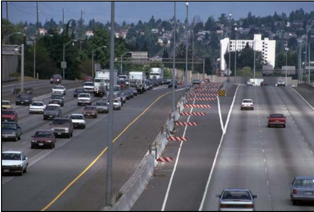
Figure 5: Ramp Gating Applied to I-5 in Seattle
