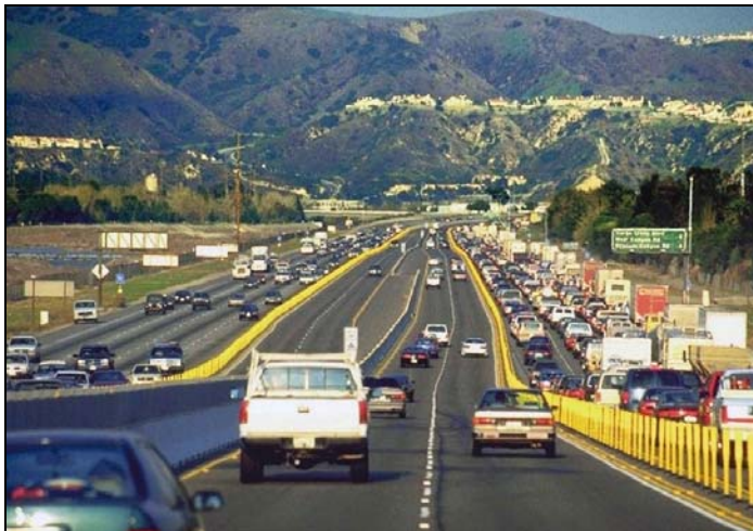
Figure 2-2: Managed Lanes on State Route 91 in California
