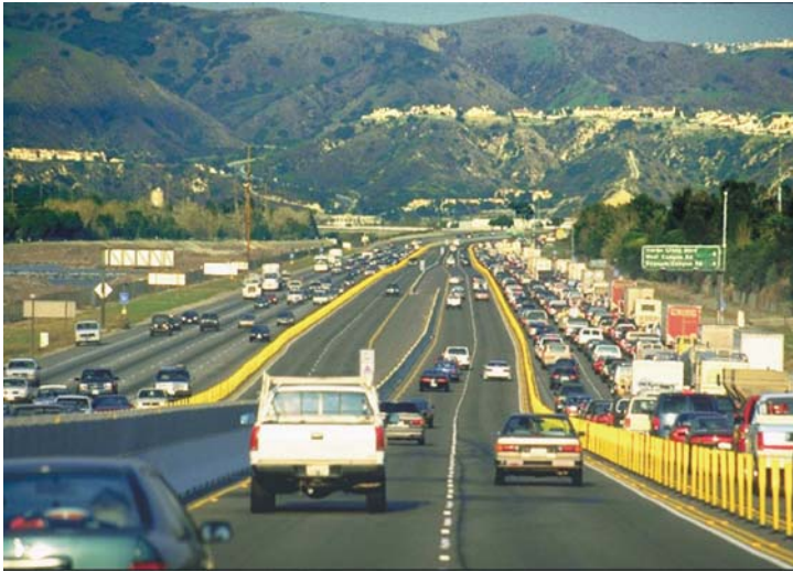
Figure 3-49: Plastic Channelizers on a Priced Managed Lanes
