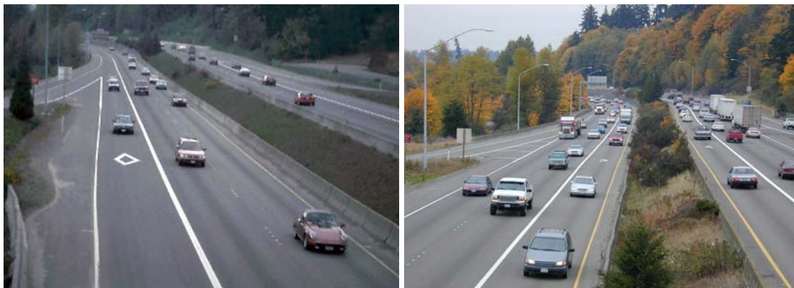
Figure 1-1: I-405 HOV Lane Before and After Conversion to Inside HOV Orientation in Seattle Area
