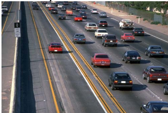
Figure 1-2: Buffer Separated HOV Lane in Southern California
