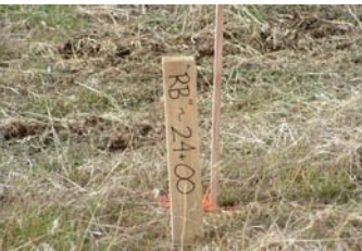
Figure 4-303.2. Slope Stake and Guinea.
