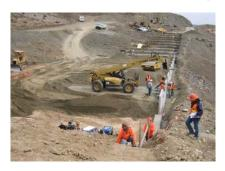
Figure 6-640.2 MSE Wall Installation.
