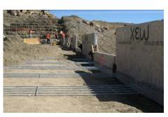
Figure 6-640.3 Soil Reinforcement Connected to MSE Wall Facing Panel.
