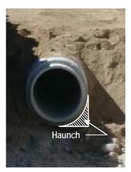
Figure 6-601.5. Pipe Backfill.
