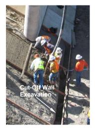
Figure 6-611.1. Slope Paving Cut-Off Wall Excavation.
