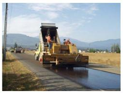
Figure 6-408.3. Chip Spreader and Hauling Trucks.
