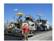
Figure 6-401.5. Plantmix Paving Machine.
