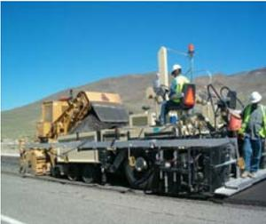
Figure 6-302.1. Class A Aggregate Base Spreader.
